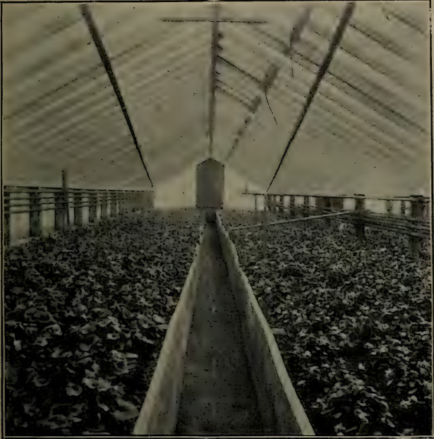
7.—House twelve feet wide, six feet to ridge; side ventilators of glass. This is one of a block of five houses, each seventy-five feet long.
